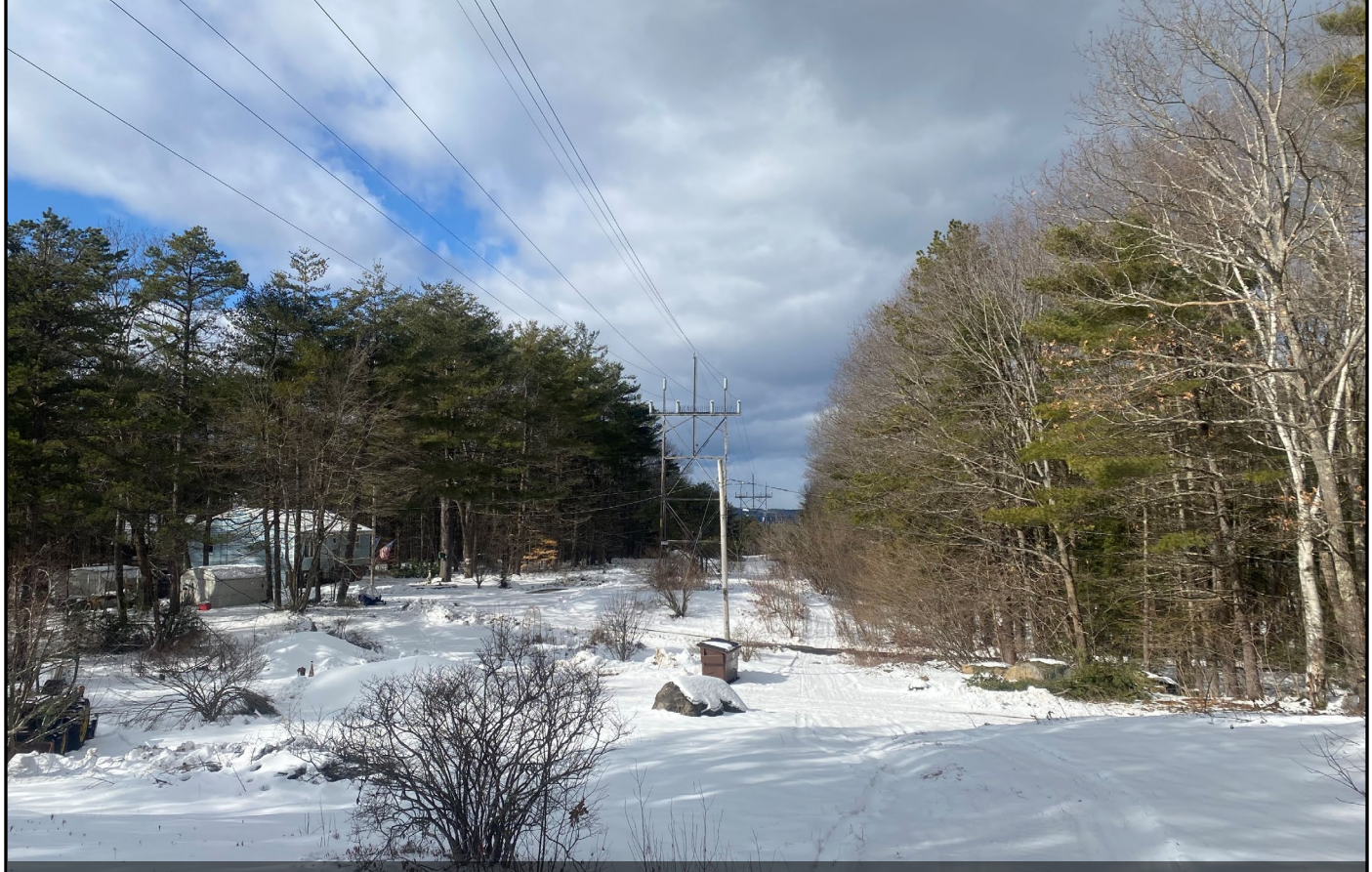
Mill Glen Road, Winchendon, MA: View 353, Existing
