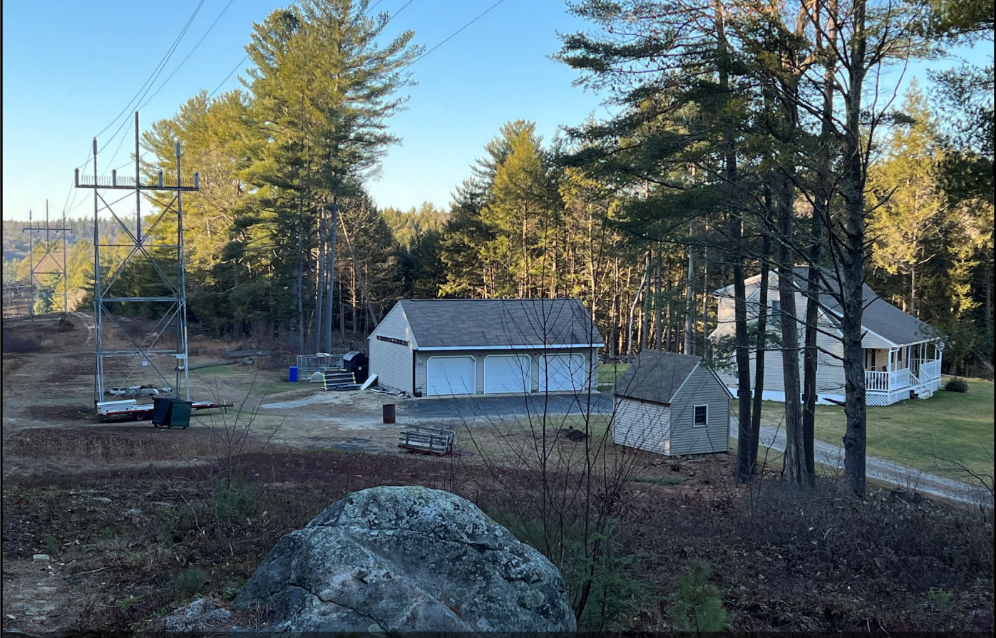
Old Winchester Rd, Warwick, MA: View 142, Existing
